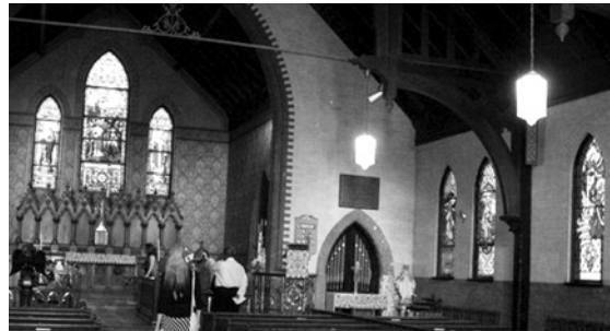
(Above) Interior view of restored stenciling surrounding altar windows
